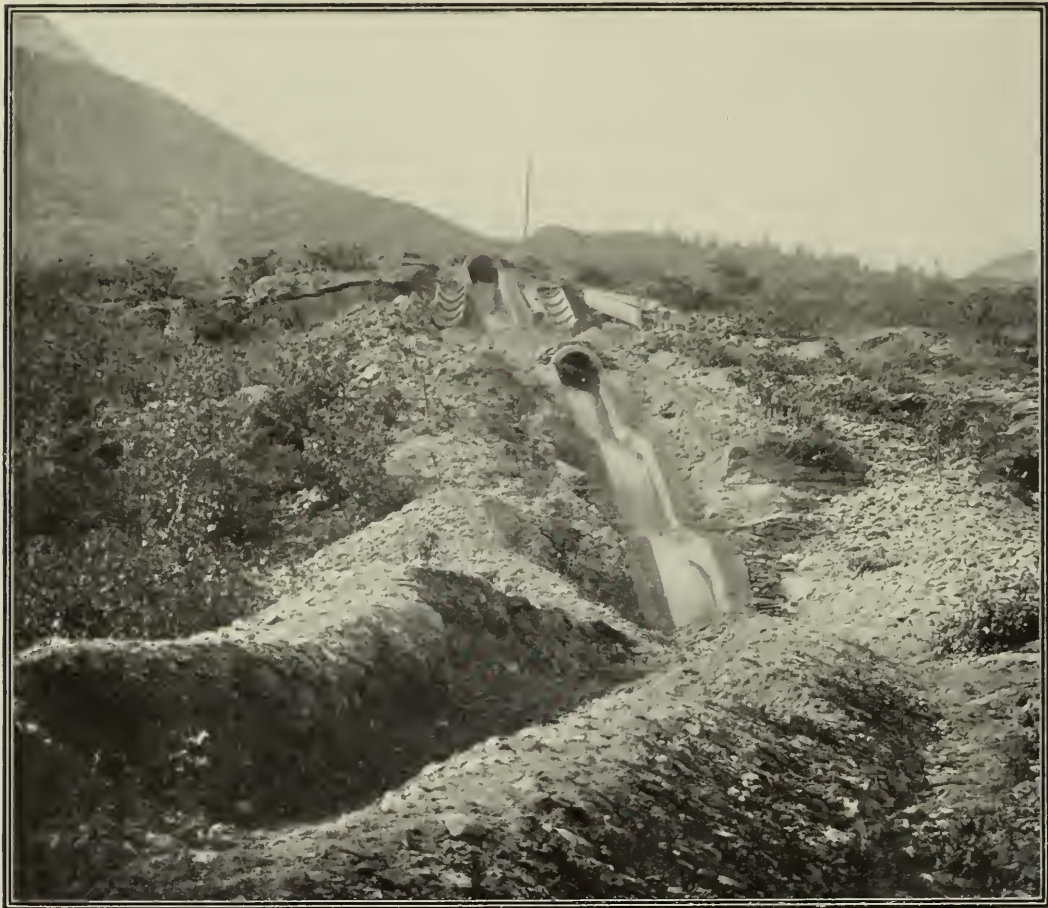
OPEN CANAL, THE PRESENT SUBSTITUTE FOR THE UPPER PENSTOCK.
